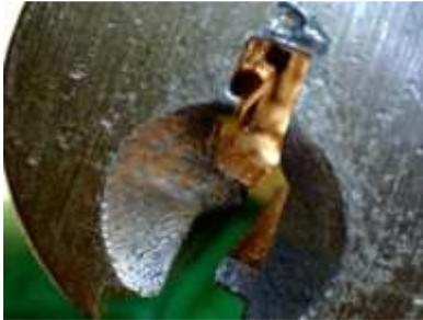
The face of a lock that has seen moderate to heavy use will have many dents and imperfections caused by normal use. How many times have you went to unlock a door and slightly missed the keyway? In the photo, many small dents and scratches from normal use are visible.
