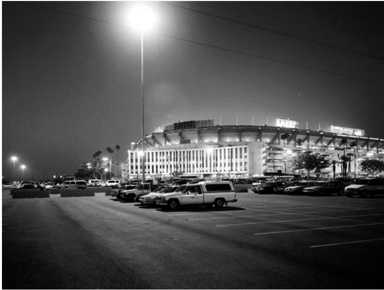
Figure 24. Parking spaces at a sports event may be some distance from the stadium resulting in long walks across parking lots. High mast HID lighting in this facility provides good horizontal and vertical illuminance for pedestrians and vehicular traffic pre- and post-game. (Photo of Holophane.)
