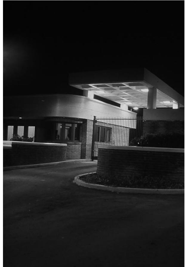
Figure 17. Driveway approach and canopy at the guard house provide uniform light for checking vehicles. (Photo courtesy of Operational Support Services, Inc.)
