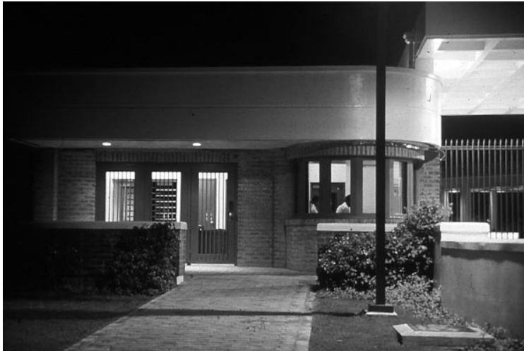
Figure 18. A well-balanced lighting system between the interior of the guardhouse and the exterior surveillance lighting. (Photos courtesy of Operational Support Services, Inc.)
