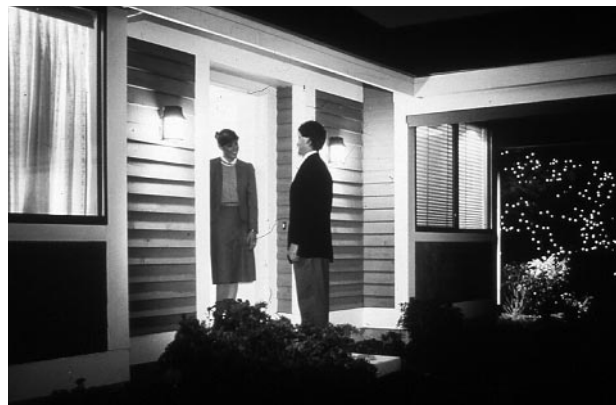
Figure 29. Luminaires mounted on either side of the door uniformly light the front door. Supplementary landscape lighting in the surrounding area contributes to a lighted welcome to visitors and enables the homeowner to easily identify the caller. (Photo courtesy of Occupational Safety Systems, Inc.)
