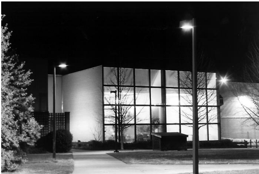
Figure 14. A combination of pole mounted area lighting units, ground mounted floodlights for building surfaces, roof mounted floodlights and an internally lit glass wall façade provide a well-lighted building environment. (Photo courtesy of General Electric Lighting Systems.)
