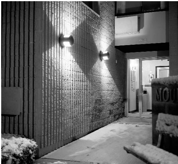
Figure 32. A well-lit entrance to a dormitory building insures safe passage for returning occupants and easy identification of arriving visitors for someone inside the building. The light distribution from wall-mounted luminaires also enhances the texture of the building surface. (Photo courtesy of Ruud Lighting.)
