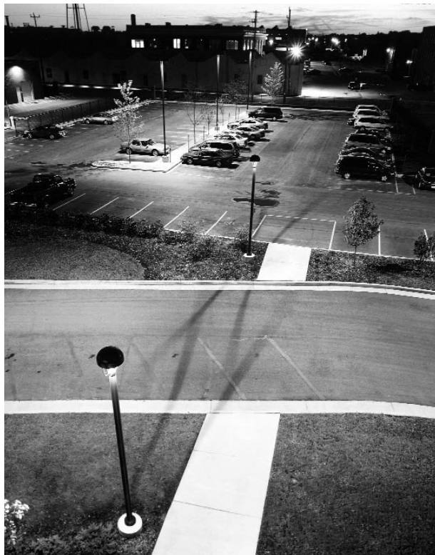
Figure 21. Cut off luminaires in an employee parking lot provide uniform illumination for workers leaving after normal business hours and excellent surveillance opportunities for observers from an upper floor in the building. (Photo courtesy of Ruud Lighting.)
