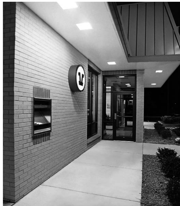
Figure 20. Recessed luminaires in the roof overhang provide uniform lighting on the walkway and vertical illuminance for customer transactions at the machine. (Photo courtesy of Ruud Lighting.)
