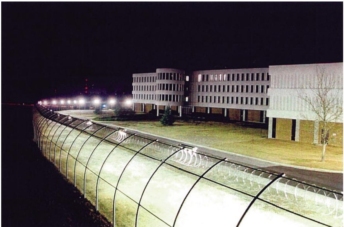
Figure 15. Instant on, reflectorized fluorescent prison lighting appears as a “wall of light” to inmates. Patrol personnel and vehicles cannot be detected during patrol. (Photo courtesy of Magnaray.)
