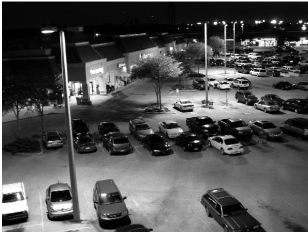
Figure 25. Parking lot lighting designed with cutoff-type luminaires not only provides a well-lighted environment for shoppers but prevents glare for drivers on adjacent roadways. (Photo courtesy of Tampa Electric Company.)
