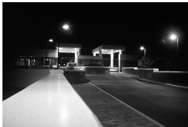
Figure 17. Driveway approach and canopy at the guard house provide uniform light for checking vehicles. (Photo courtesy of Operational Support Services, Inc.)
