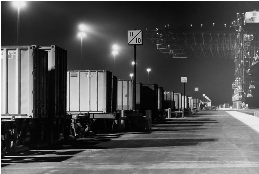
Figure 13. Container storage yard is uniformly lit with good vertical illuminance between the containers. (Photo courtesy of General Electric Lighting Systems.)
