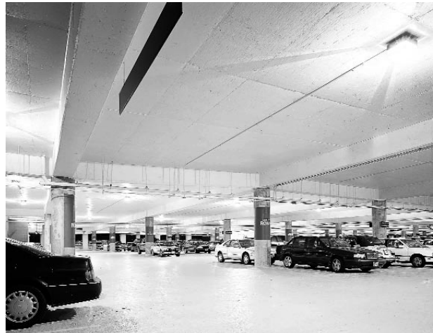
Figure 23 (b). A higher ceiling and light surfaces throughout results in a uniform distribution of light and a shadow-free environment. (Photo courtesy of Ruud Lighting.)
