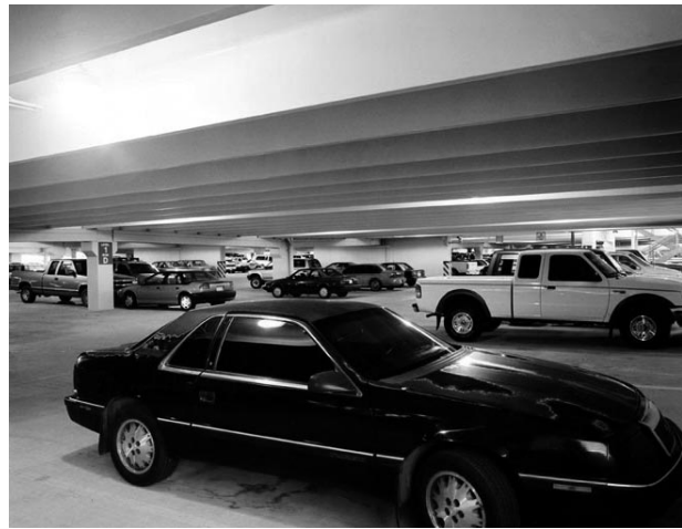
Figure 23 (a). Structural elements afford concealment of luminaires. When coupled with a low ceiling, the designer may be challenged (successfully in this case) to provide uniform lighting in the space, especially between parked cars. (Photo courtesy of Holophane.)
