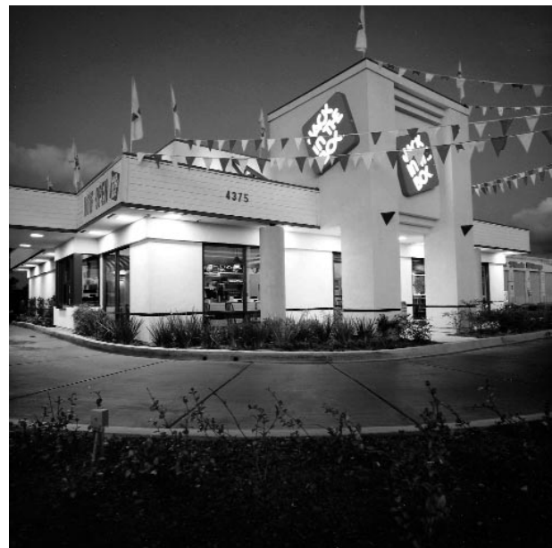
Figure 26 (b). Recessed luminaires define the building with a soft wash of light and highlight the drive-up window, allowing window-service personnel to clearly see the arriving customers. Light surfaces reflect light onto the driveway for easy way-finding. (Photo courtesy of Ruud Lighting.)
