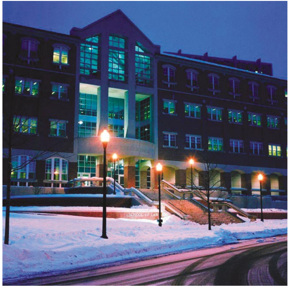
Figure 34. Lighting for vehicular and pedestrian traffic facilitates surveillance when security issues are a high priority on campus. (Photo courtesy of Holophane.)
