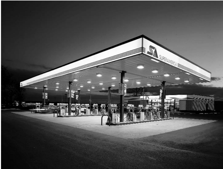
Figure 27 (b). Well-balanced horizontal and vertical illuminance insures safe and secure task performance at the pump island and visibility of outdoor areas to people inside the store. (Photo courtesy of Ruud Lighting.)
