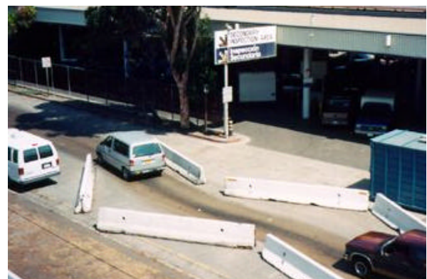
Figure 7. Concrete Delay Barriers
