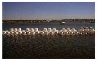
Marina on Sodus Bay in Lake Ontario, New York we are showing a transmission coefficient of 0.1 on the expected wave spectrum. The Marine Barrier was able to dissipate the 4foot waves that the marina was subject to during highly destructive storms to a mere 6 inches (90% efficient)!
