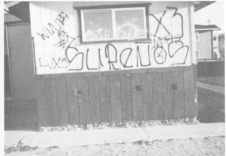
The graffiti on this apartment building in Carson City, Nevada, identifies the gang members who claim that turf as being from Southern California.
