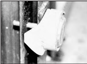
(Above) American 2000 lock with shield and pin.
