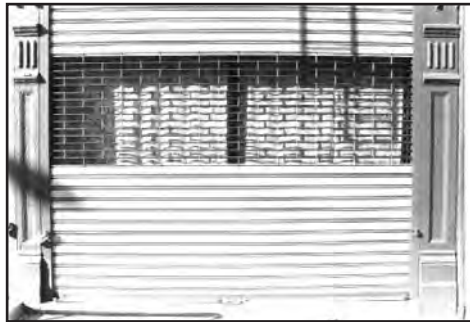
(Above) A combination gate with steel interlocking slats on the top and bottom and an open grill in the center. This gate is operated manually.
