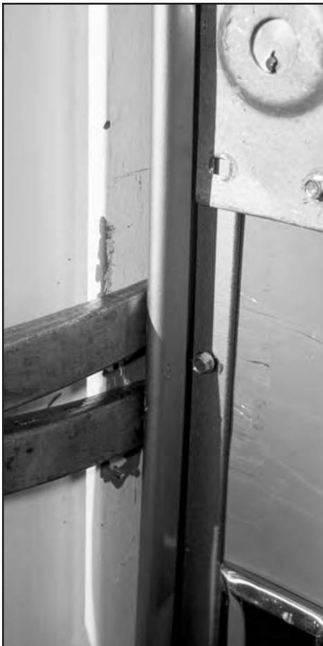
Figure #9--A newer type of device is an angle iron with a metal, J-shaped shield screwed into the door frame.
